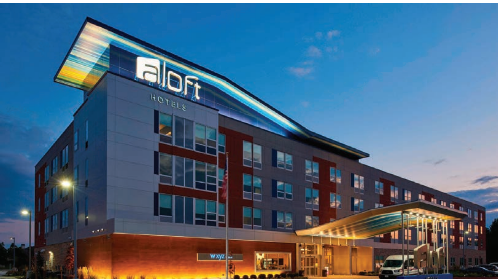
ALOFT CLEVELAND AIRPORT EXTERIOR
