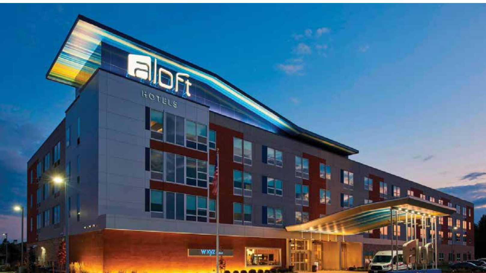
ALOFT CLEVELAND AIRPORT EXTERIOR
